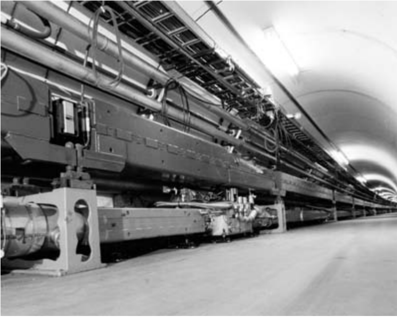
10.1 Interior of the Main Ring with the ring of superconducting Energy Doubler magnets below the original ring of conventional magnets, 1983. (Courtesy of FNAL Visual Media Services.)
