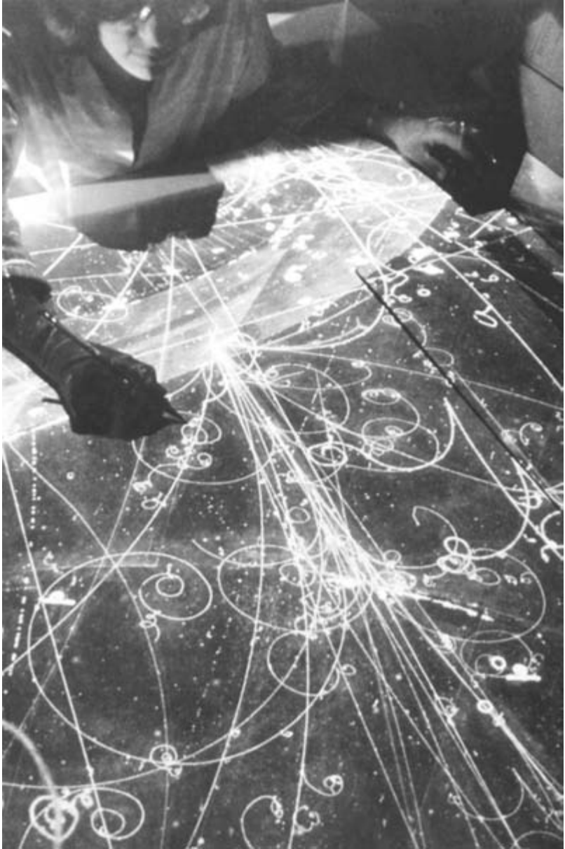
7.2 Scanner looking for unusual particle interactions in a bubble chamber experiment photograph, 1978. (Courtesy of FNAL Visual Media Services.)
